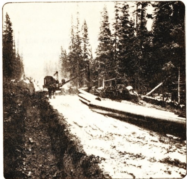
Construction on the Silver Dohl Pipeline.
