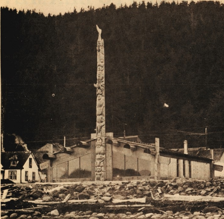
Skidegate Band Administration Building Photo: C. Linde
