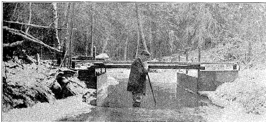
Measuring Flume on Josephs Creek, near Cranbrook.
