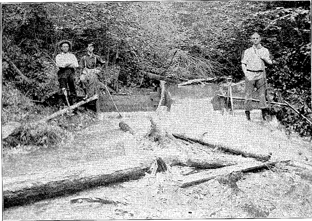
Cippoletti Weir, Maguire Creek, during construction.
